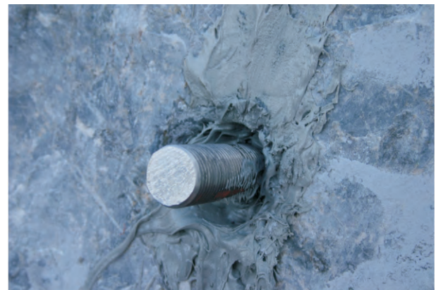
Offset in rock anchor shell with anchor rod
